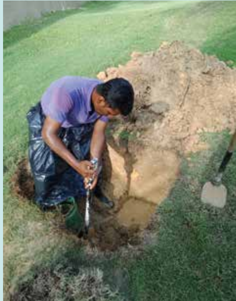
Sprinklers repair underway at West 3 course
